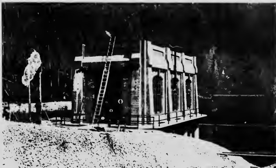
Coquitlam-Buntzen Development. Intake Valve House, Plant No. 2, looking towards Lake Buntzen.
